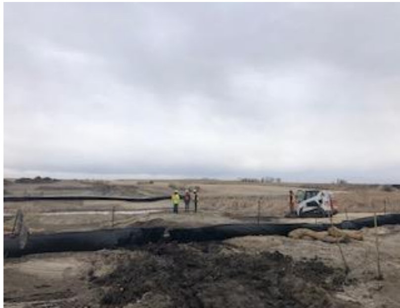
Sediment removal with skid steer
