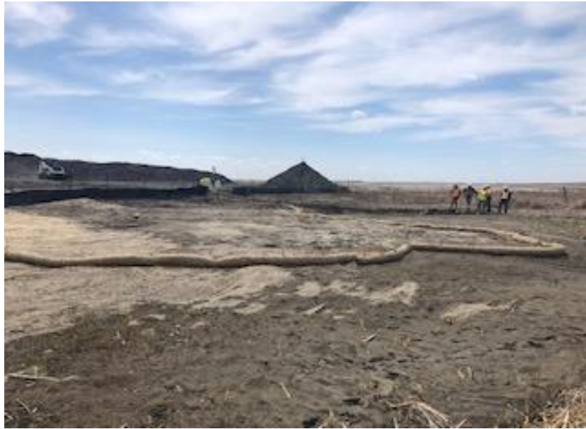
Water course crossing clean-up
