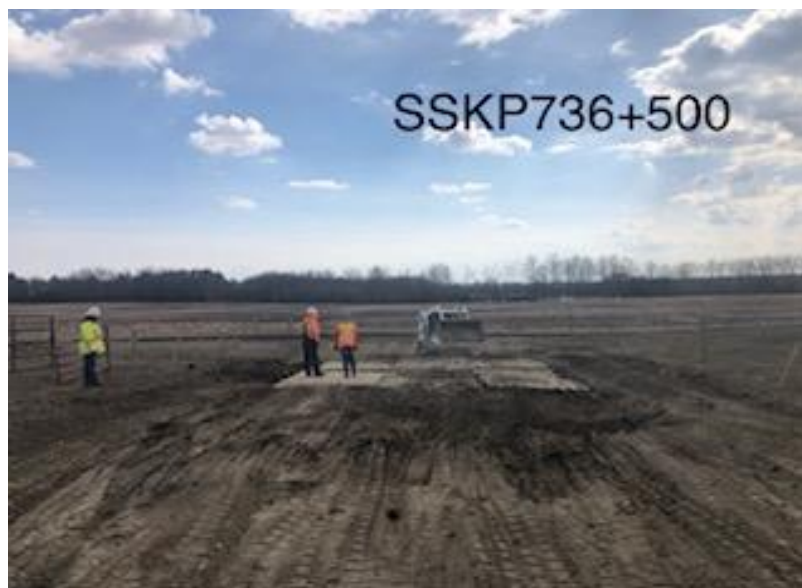
Mat installation at SF801
