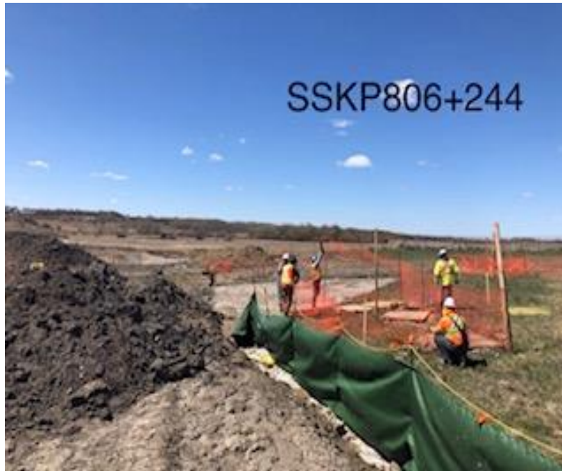
Snow fence repair
