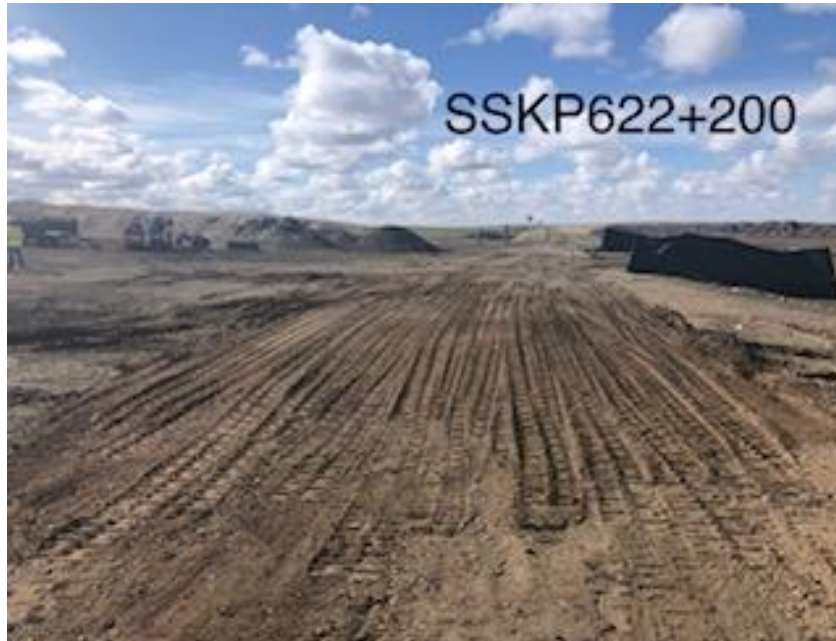
Access plug being repaired
